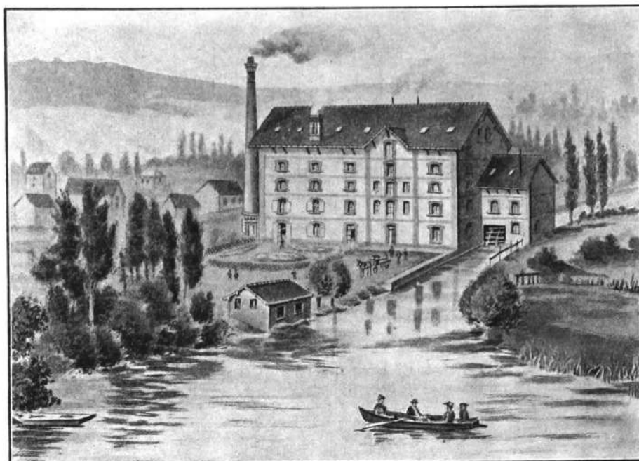
Couesnon & Cie. Clarinet Factory at Garennes, France
