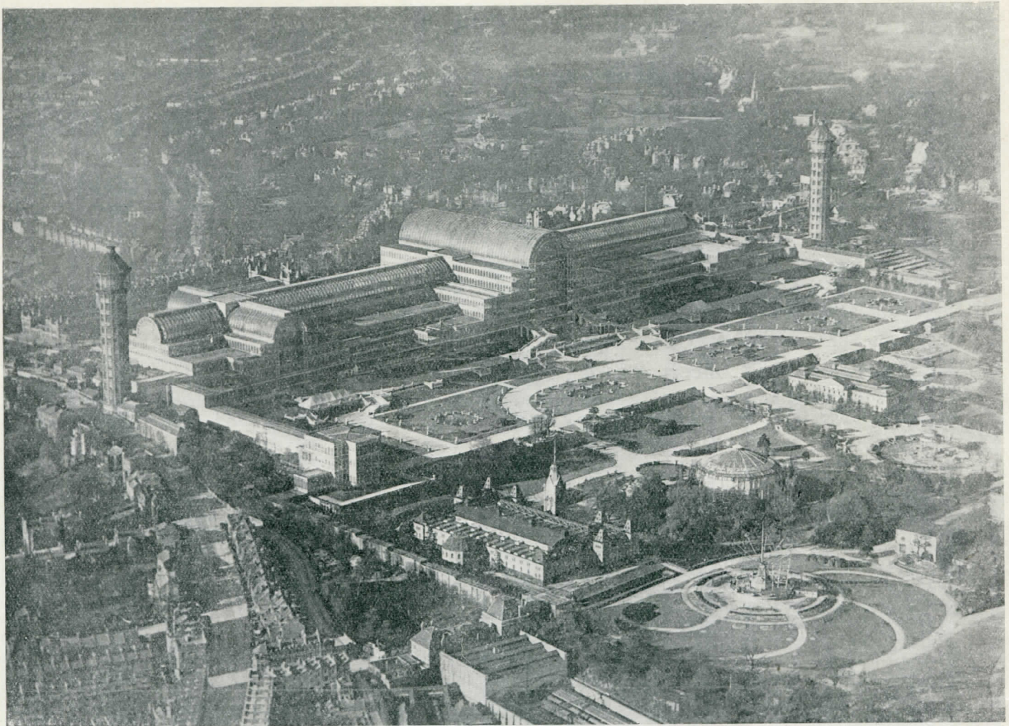
AERIAL VIEW OF CRYSTAL PALACE
