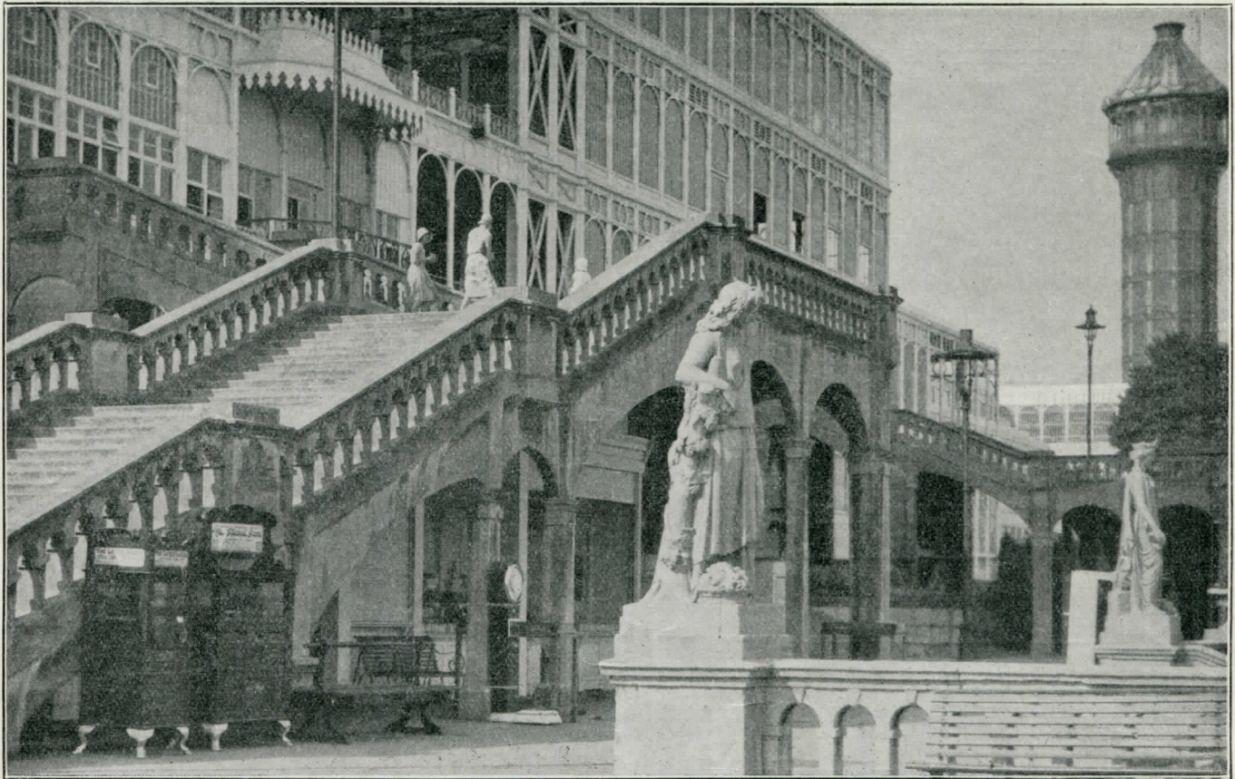
LOOKING TOWARDS THE GRAND STAIRWAY, CRYSTAL PALACE
