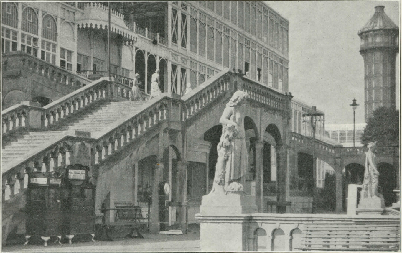
LOOKING TOWARDS THE GRAND STAIRWAY, CRYSTAL PALACE
