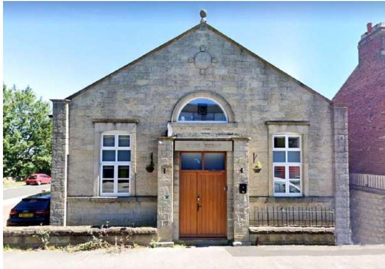
Grove Park Methodist Chapel
